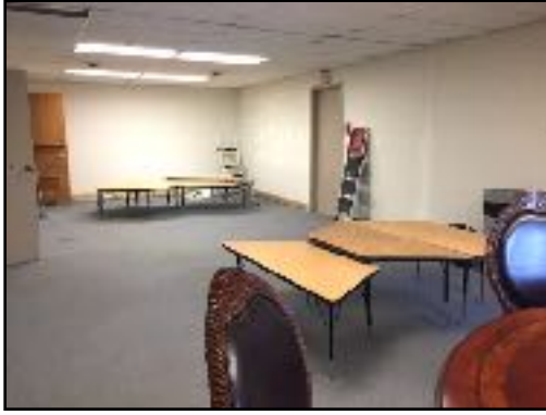
The results of the work of Nancy Herrington and Abbey Aymes can be seen in this photo of rooms 4 & 5. The folding room divider and wall cabinets have been removed and the walls scraped, cleaned, and spackled. All is ready for painting and carpeting.
